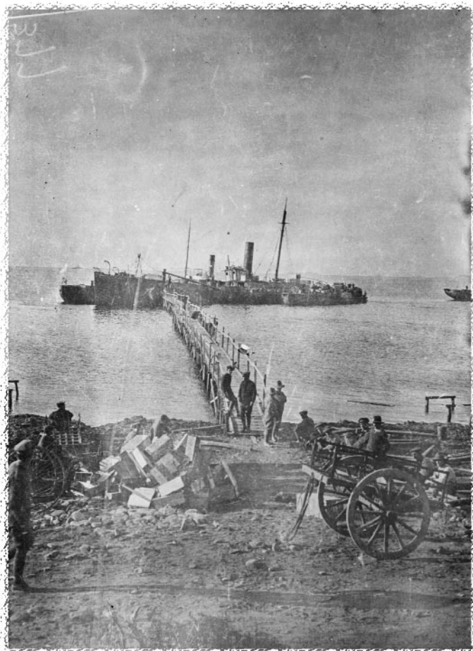
Shortly before the final evacuation of Anzac, Australian engineers built a wooden walkway out to the beached steamer Milo, which had shifted slightly away from Williams' Pier in the November storms. Many Anzacs were evacuated from this temporary pier. (AWM A01032)
